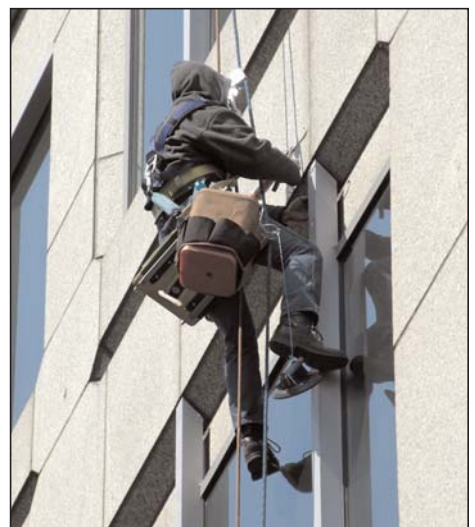
Until it was banned in 1997, PCB had been used in building caulk
