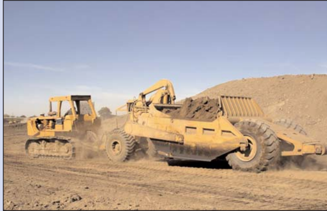
Earth-moving equipment breaks ground for new development.
