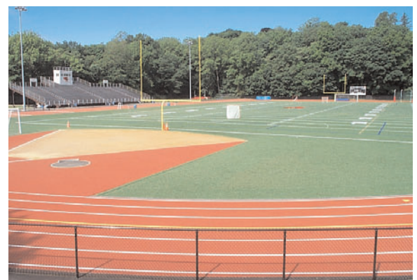
End-zone view of new synthetic track and field with shotput event shown, Greenwich High School, Greenwich, Connecticut.
